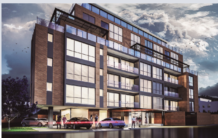
Verona, Cuenca. General view of the building
