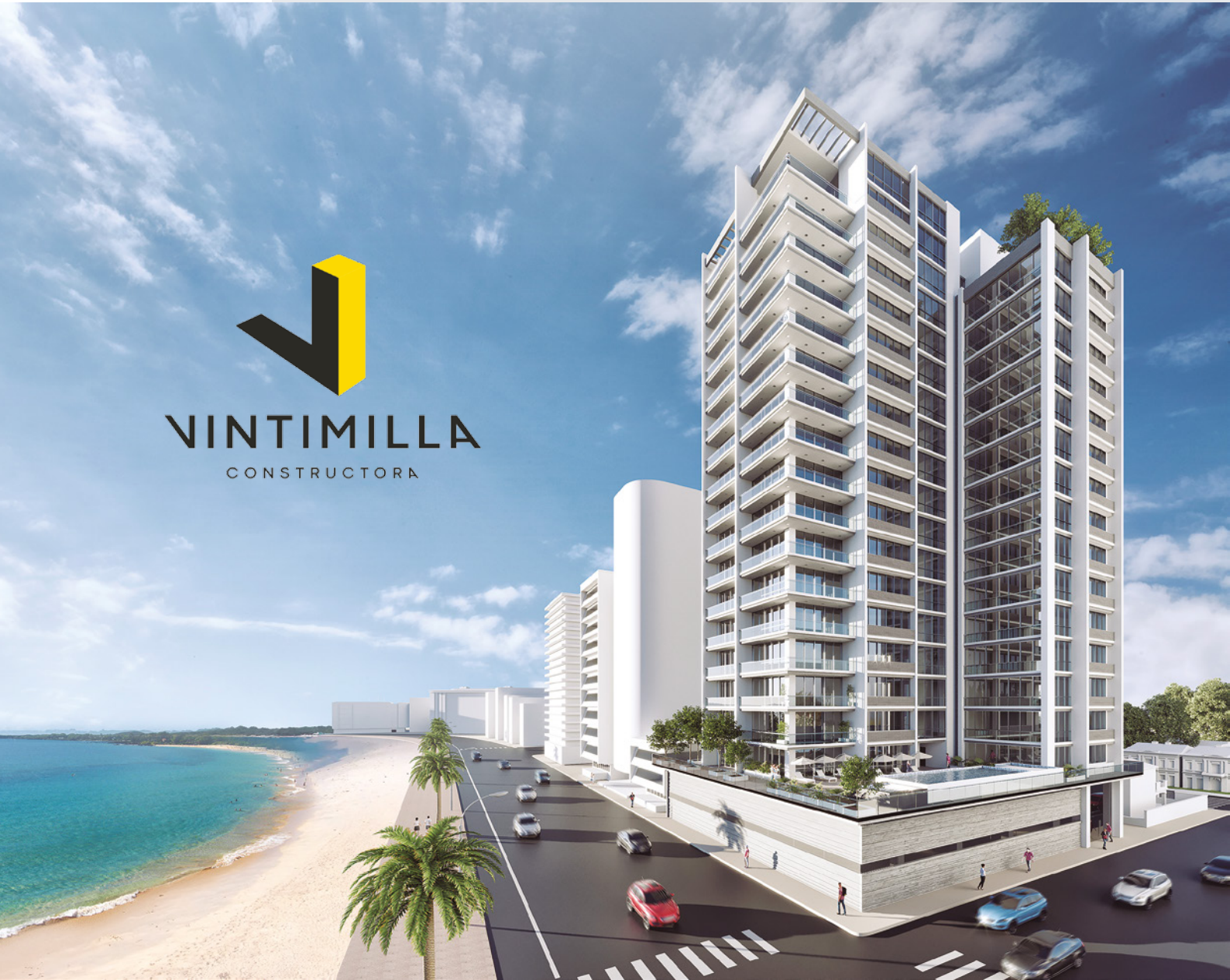
Perla Azul, Salinas. General view of the building
