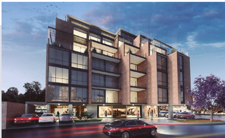
Verona, Cuenca. General view of the building
