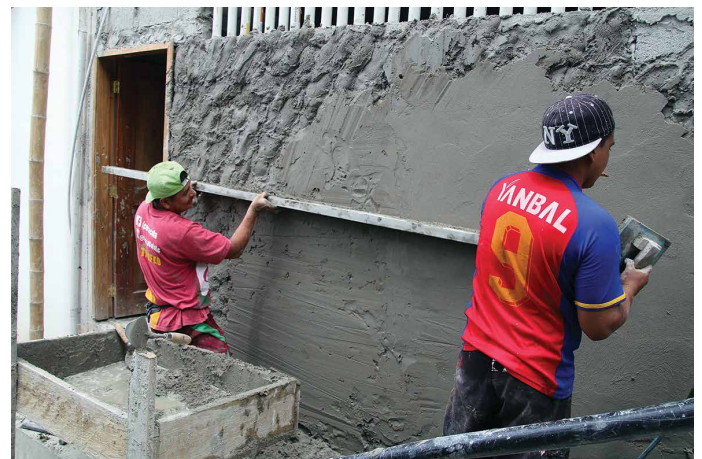
Repairs are part of the plan to colorize the village
